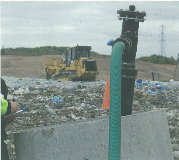
Gas extraction chamber
