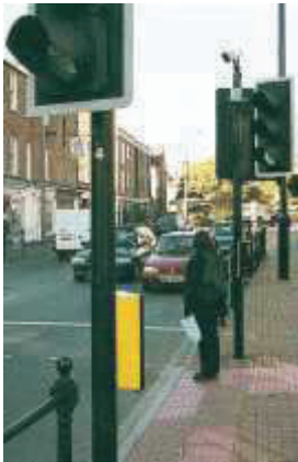
Typical layout of a Puffin crossing showing the detectors and offset mounted traffic signal ahead
